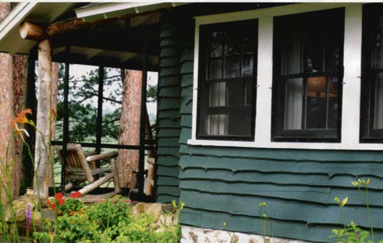
White Pine Camp, in Paul Smiths, the first documented site of brainstorm siding in North America. Photograph by Kelly Hogg
